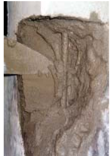
Apply the mortar
