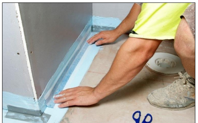
Installing Elastoproof B50 Bond Breaker Joint Band
