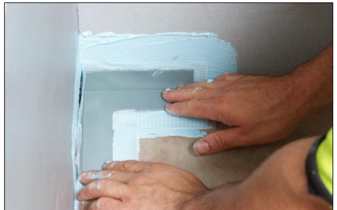
Installing Elastoproof Prefabricated Corners
