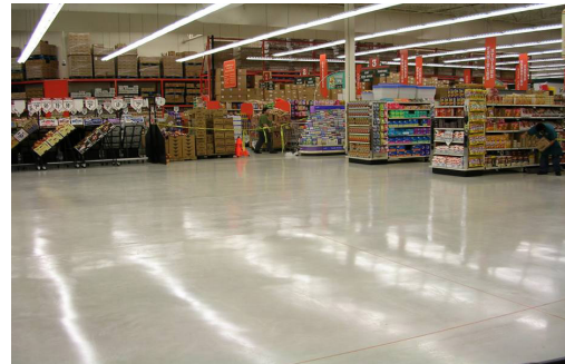
Typical steel trowel finished concrete with one coat of Durafloor HD and three coats of Durafloor HD-S.
